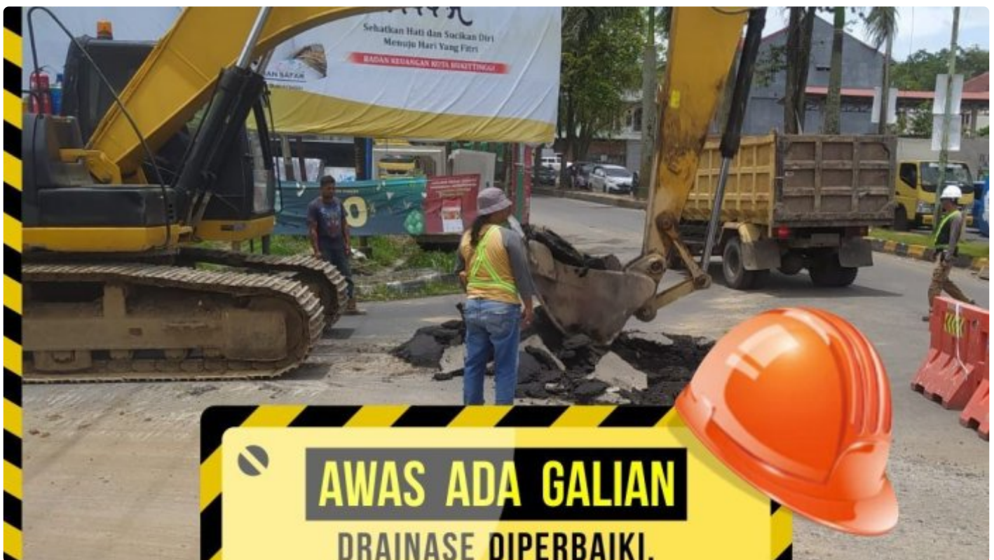
Drainase Diperbaiki, Upaya Pengendalian Banjir By Pass Bukittinggi
